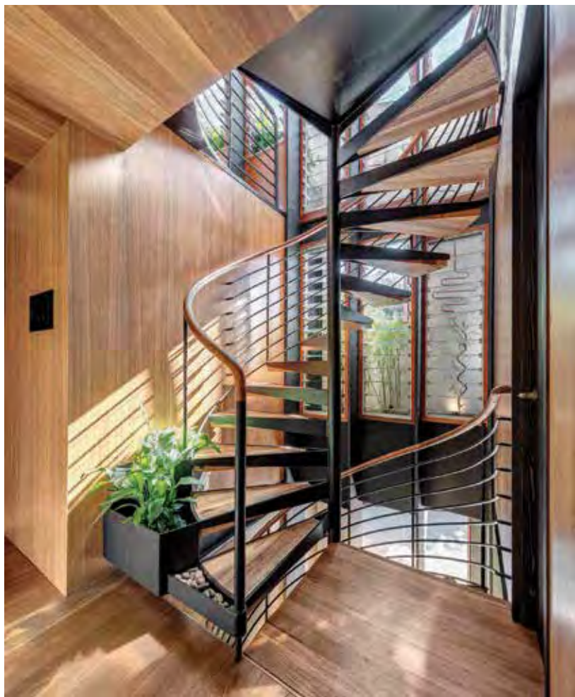
top left A large pivoting shutter allows for light and ventilation when open or closed. right Bunk beds and cupboards are all built in. bottom left The spiral staircase flushes out hot air through the north-facing louvre windows. right Original openings are framed with pre-rusted steel, and new openings with white powder-coat steel.
