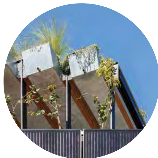
Steel troughs have native plants and a productive garden, as well as clay beads that grow bacteria to filter water.
